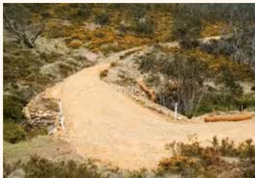
Stockyard Creek crossing on the upgraded section of Mt Franklin Road.
