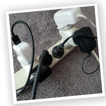
Overloaded power points and power boards can overheat and cause a fire in your home.
